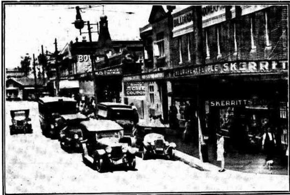
Figure 15 – Good Street, Granville looking south from Sydney (Parramatta) Road. 36-42 Good Street on right with Turret of Patten's building clearly visible beyond and the enlarged Fire Station in between. (Source: Cumberland Argus and Fruitgrowers Advocate, 12 December 1929, p2)
