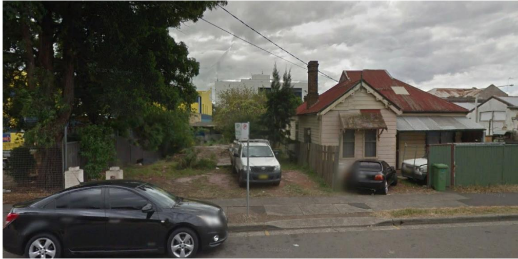
Figure 20 - Sites in Cowper Street showing the surviving timber cottage at 59 Cowper Street and the site of demolished buildings adjoining at 61 Cowper Street
